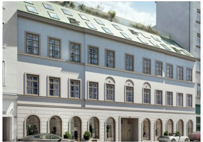
The Fusion | Fassade
