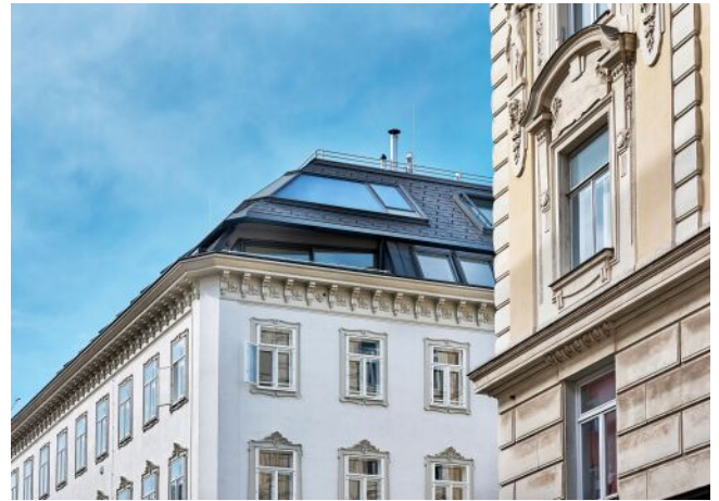
Essenz No. 1 | Fassade
