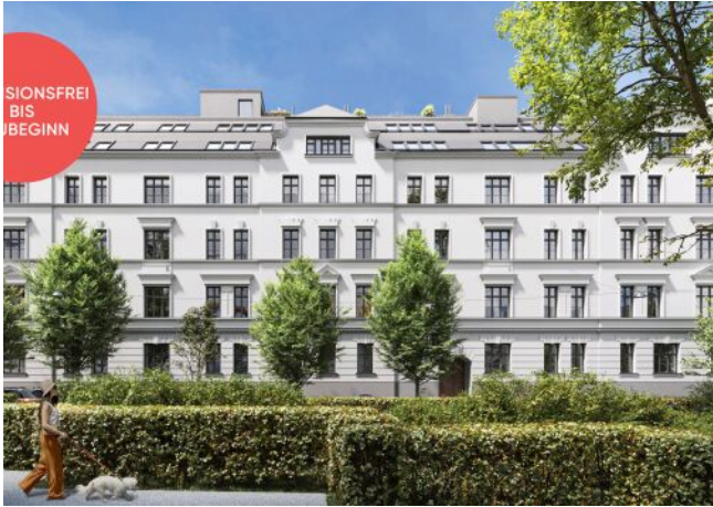
Roseggergasse | Fassade Frontal
