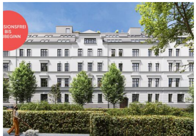
Roseggergasse | Fassade Frontal
