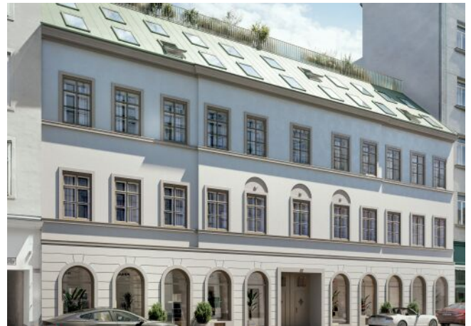
The Fusion | Fassade
