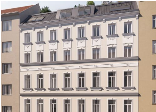
The Core | Fassade Tag
