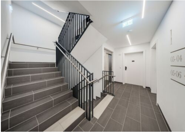
The Unique Apartments | Stiegenhaus
