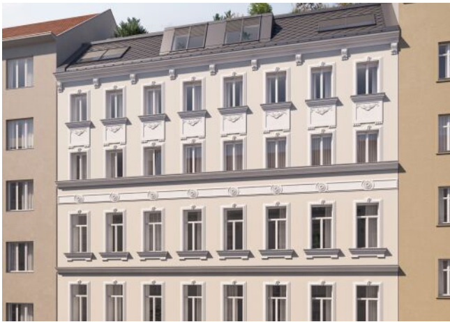
The Core | Fassade Tag
