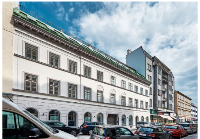
The Fusion | Fassade
