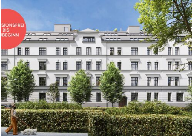
Roseggergasse | Fassade Frontal
