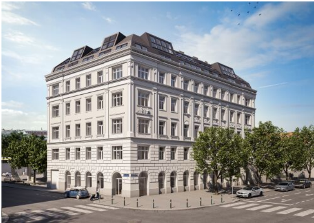
The Legacy | Fassade
