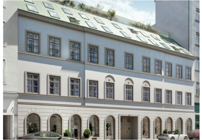
The Fusion | Fassade
