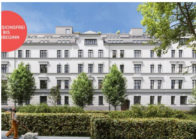
Roseggergasse | Fassade Frontal
