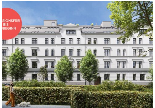
Roseggergasse | Fassade Frontal
