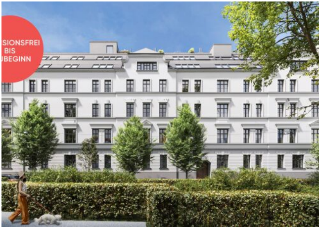
Roseggergasse | Fassade Frontal
