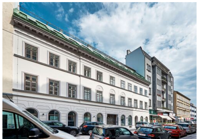
The Fusion | Fassade
